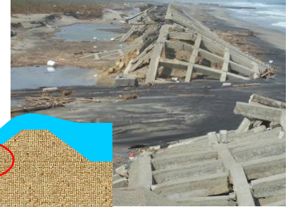
Embankment destroyed by TSUNAMI
